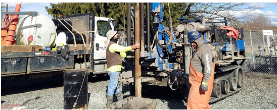
Example of a drill rig used for geotechnical boring.
